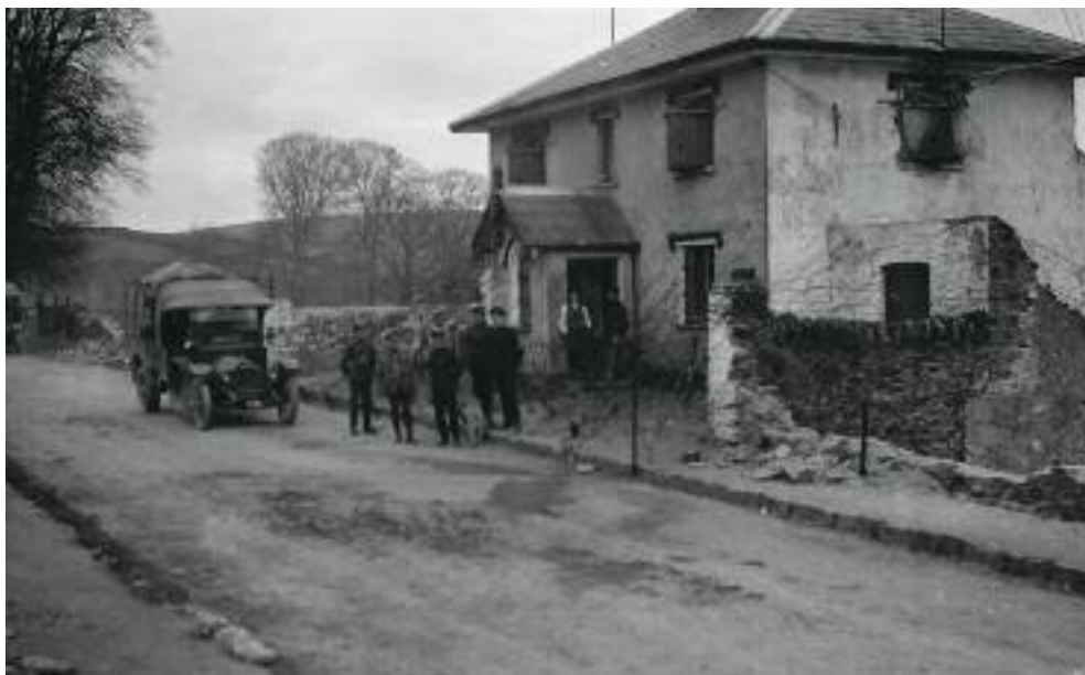
In an effort to defend the RIC barracks, their defences were augmented, particularly with the addition of armour plating over entry points like windows, as can be seen with this example at Ballinhassig.
